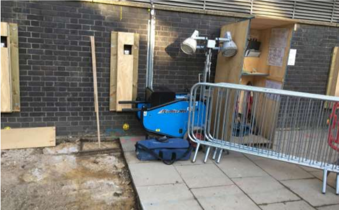
Hydrogen tower lights
