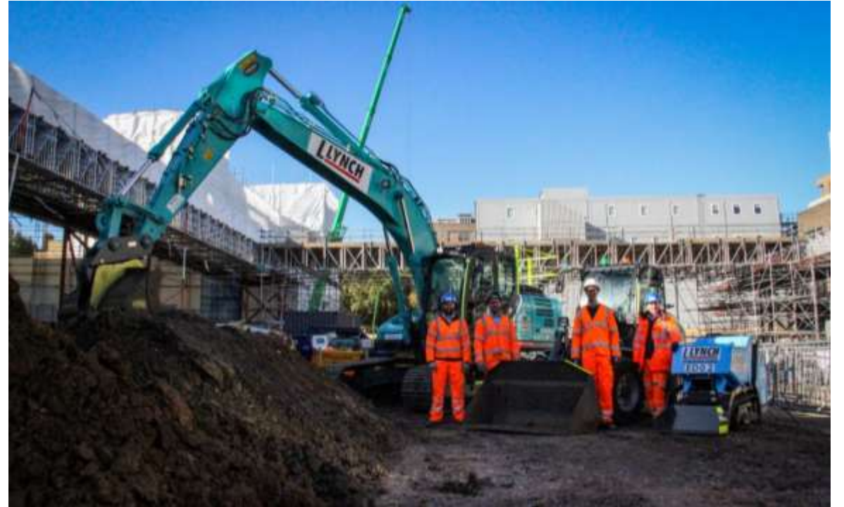
Hybrid Excavator & Electric Wheelbarrow
