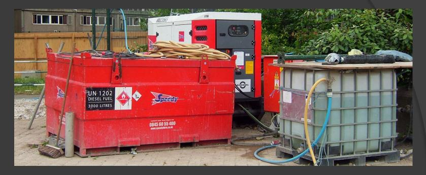
Trial to assess the impact of using smart generators which automatically sense the load on a diesel generator and switches between battery power and diesel power accordingly.
