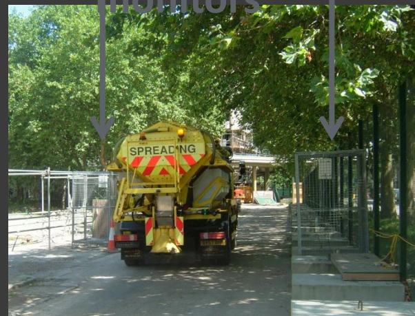
Application dust suppressant
